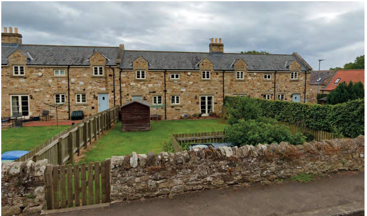
Recent development in Rock showing attention to detail reflecting local character.
