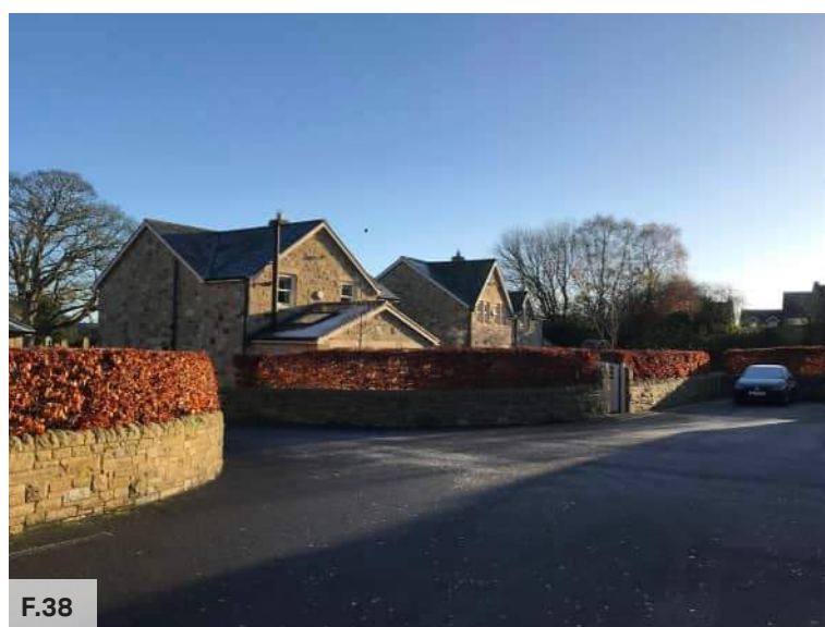
Figure 38: View of the rear of 1 & 2 Church View and their low sandstone walls
