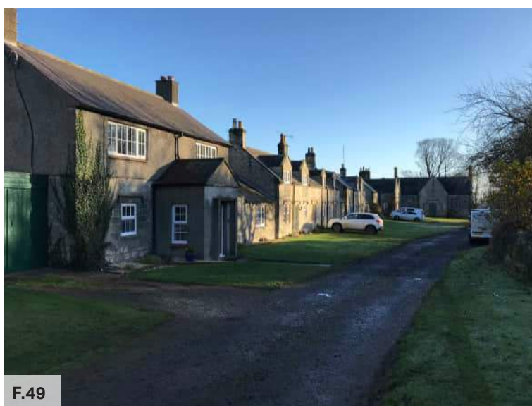
Figure 49: View of the access road
