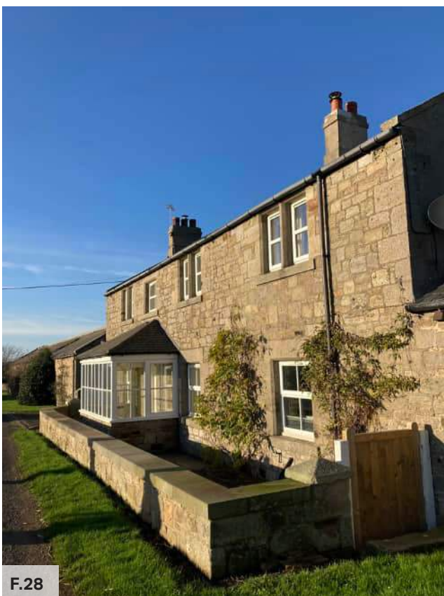
Figure 28: Low sandstone boundary walls are a frequent boundary treatment in the area
