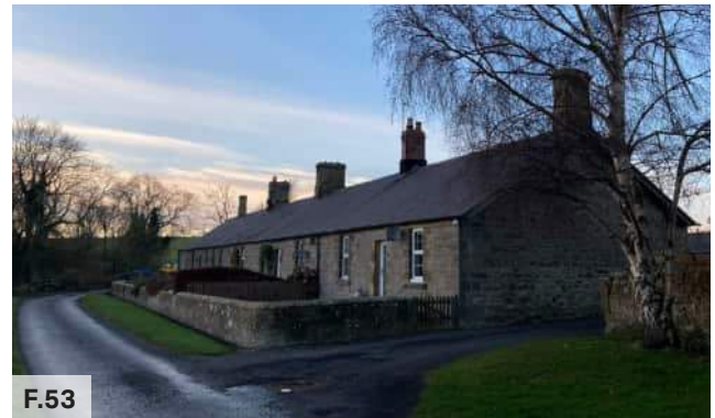
Figure 53: Terraces following road alignment in Rennington village
