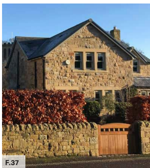
Figure 37: View of the rear of 3 Church View
