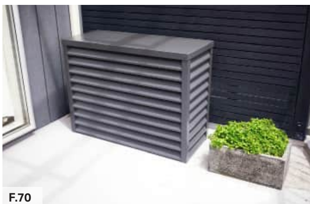
Figure 70: Air source heat pump housing covers the unit and harmonises with the building aesthetic
