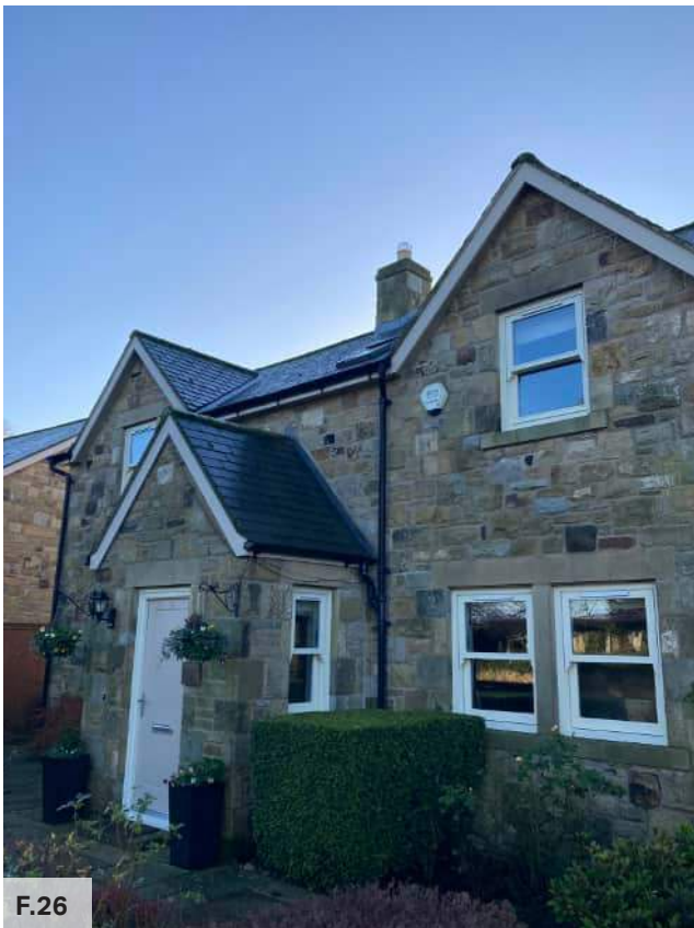
Figure 26: Windows often have lintels, architraves or quoins in the Neighbourhood plan area
