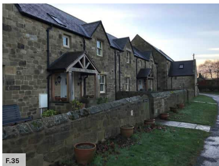
Figure 35: View of the terraces including their front gardens and low sandstone walls
