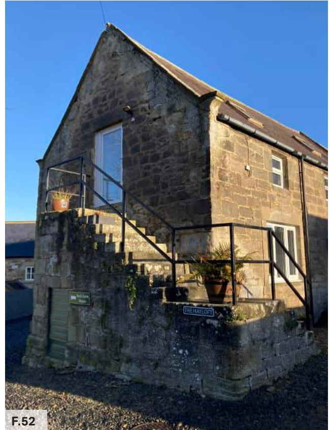
Figure 52: Sandstone building in Rock village
