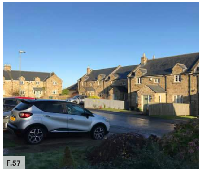
Figure 57: Internal service area Rock Home Farm
